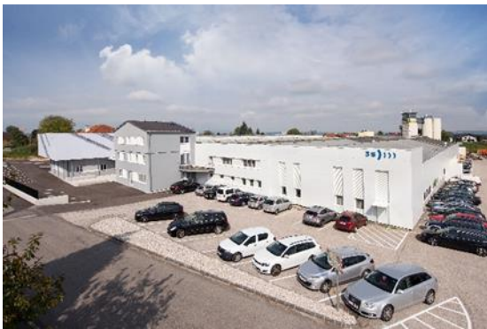
Photo 1: At the company headquarters in Roitham, 3S expanded production area and company headquarters.
